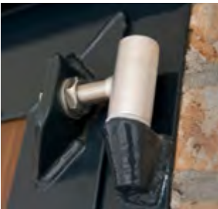
Adjustable hinges made of stainless steel
