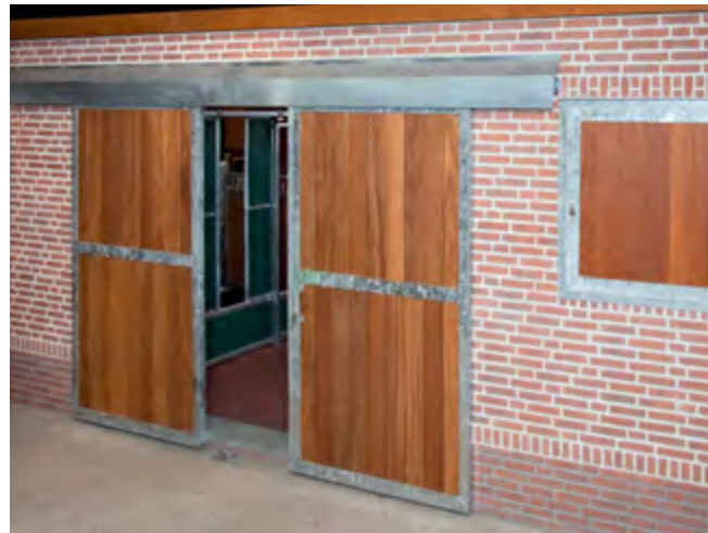
Vertically divided double sliding door with cover strip over guide rail
