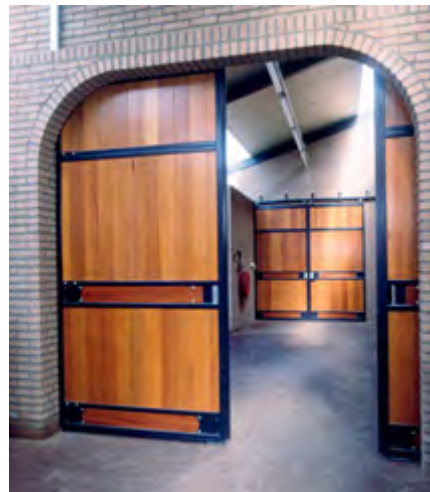
Custom made double sliding door which slides into a wall cavity. A particularly beautiful visual effect is created by the rounded brick arch.
