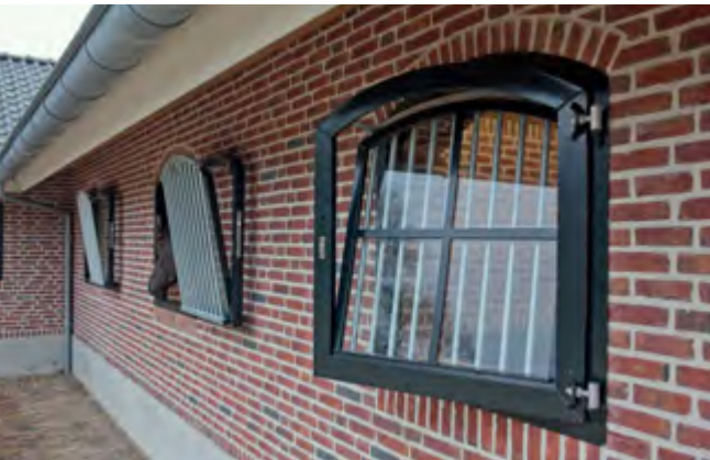
Turn-tilt system with additional protective steel spindles (galvanized), frame powder-coated, additional rungs as decorative element
