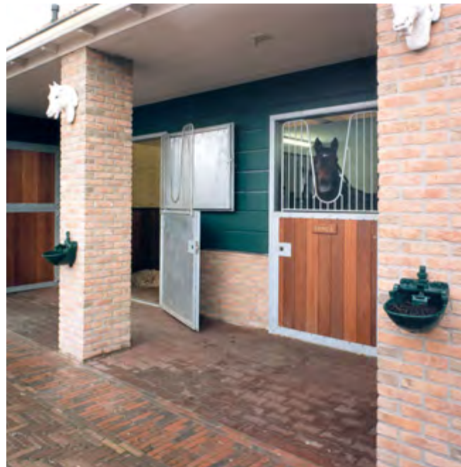
Stall doors with tread and bite guards on the inside and V-grid insert in the upper part
