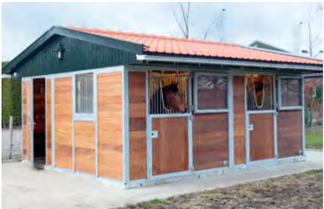
Exterior stables with 12° gable roof, interior stalls and aisle
