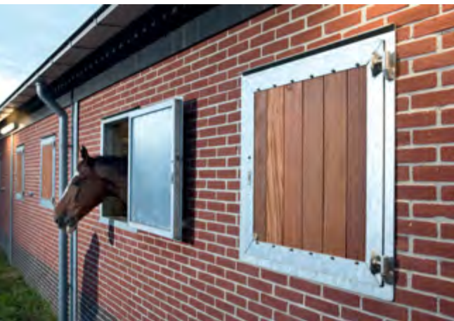
Professional window with wooden planks on the outside and bite guard on the inside
